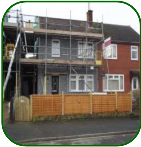
External Wall Insulation in Hucclecote
